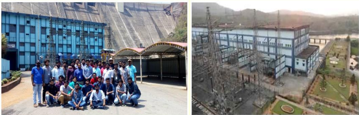
Figure 7 Supa Power house Dandeli , Supa Power grid system Dandeli
